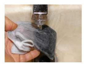
Slip the bag into the filter housing, fold the rest of the bag down on top.
